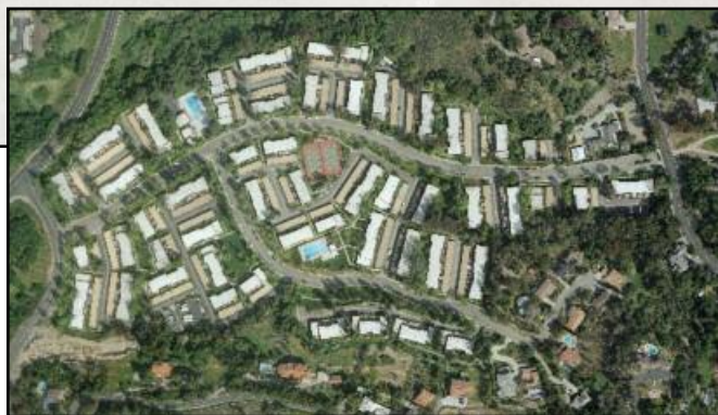
THE NEW ROOF ON THE TIBURON PUDDINGSTONE TOWNHOMES IN SAN DIMAS, CALIF. BELOW, AN AERIAL PHOTO OF THE PROJECT.
